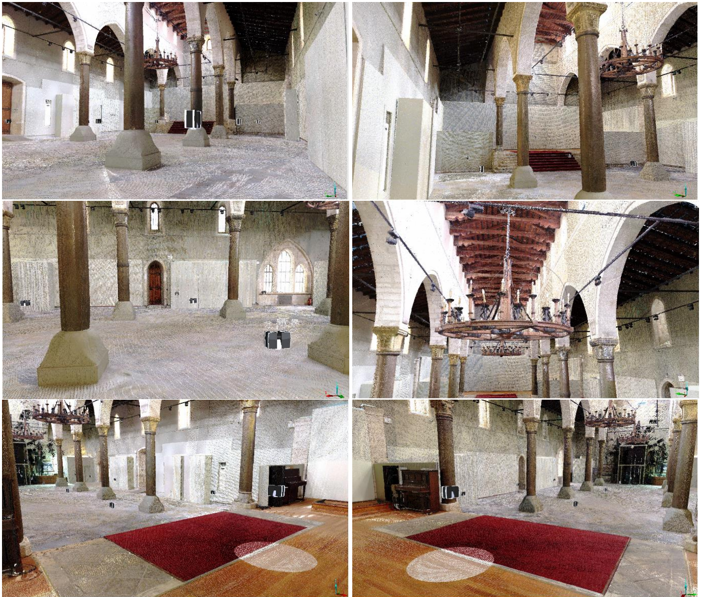
Figure 4. Registered 3D point cloud.
